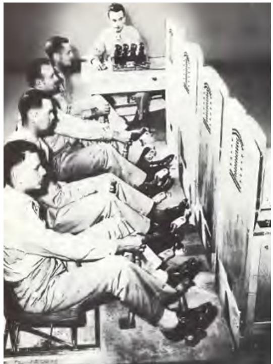
Figure 3. This U.S. Air Force photo shows four examinees taking the Complex Coordinator test, which was used for pilot selection. Examinees controlled a hand-stick and a rudder bar (using their feet) while monitoring a display board that had three sets of two lines of light bulbs (one green, the other red; Munn, 1962). The examinees used these controls to move the green lights and match them to three lit red lights.
